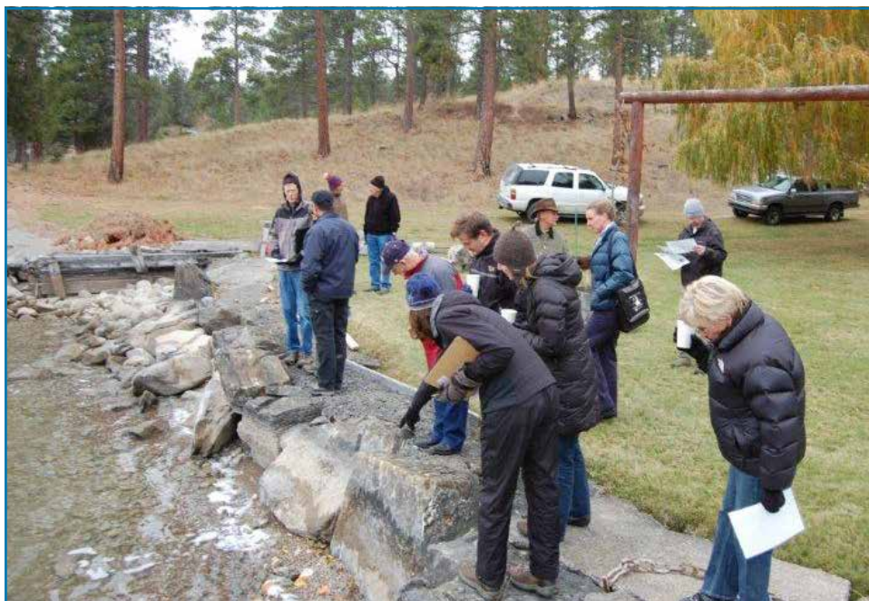
Walk & Talk Tour participants examine the crumbling sea wall that will be replaced with a more natural shoreline when the vegetated buffer is planted on this property. photo by Laney Hanzel
