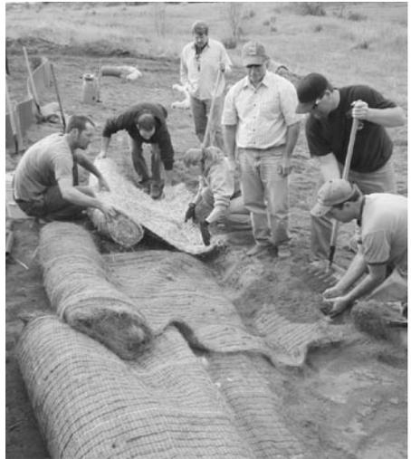
**Participants in the Stormwater Erosion Education Program class learned how to correctly install erosion control blankets that help prevent erosion during construction projects. photo by Constanza von der Pahlen**
